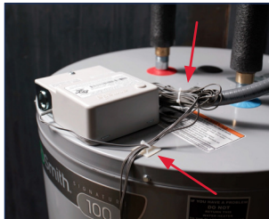
Figure 31 - Excess Wires
