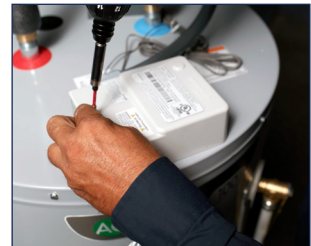
Figure 24 - Tighten Top Screw
